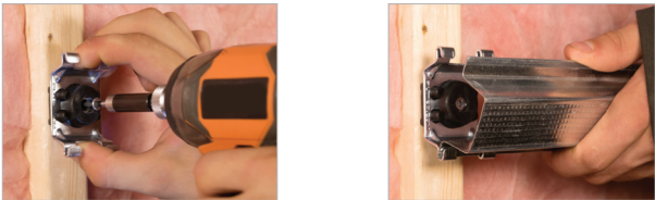
Figure 7: Installation of Pliteq GenieClip RST
