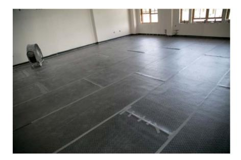
7. Use **GenieMat® PMI** to wrap all columns, drains, penetrations to ensure there is no hard surface contact with the topping material (plywood or concrete).
