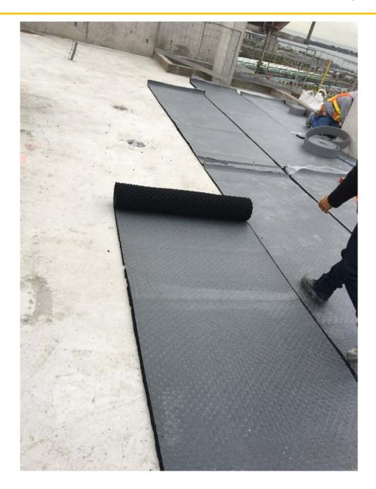
6. Use duct tape or high-quality carpet tape to secure butt joints and seams, and prevent underlayment from moving. If multiple layers of GenieMat FF are being used (i.e. **GenieMat FF50**) then only the seams on the top layer need to be taped.
