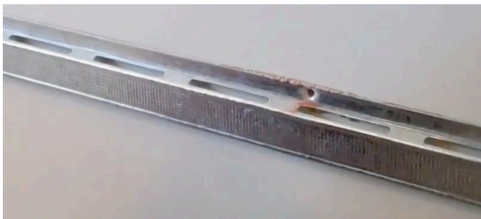
Figure 4: Still image from a how-to video 5 that shows RC being installed incorrectly
